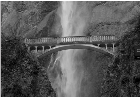
FIGURE AP-22 The image after the brushwork on bridge for lightening
